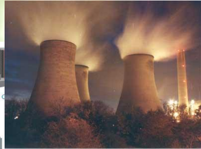
Coal-fired power station ~ 30-35% efficiency
